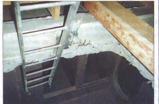
A thick layer of concrete had to be breached to provide a new stairwell.
